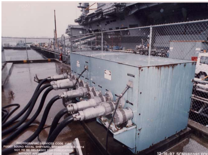
Figure 13-8. 4.16 kV Pier Electrical Outlet Assembly and Outlets
