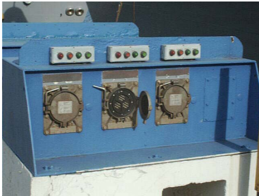
Figure 13-8. 4.16 kV Pier Electrical Outlet Assembly and Outlets
